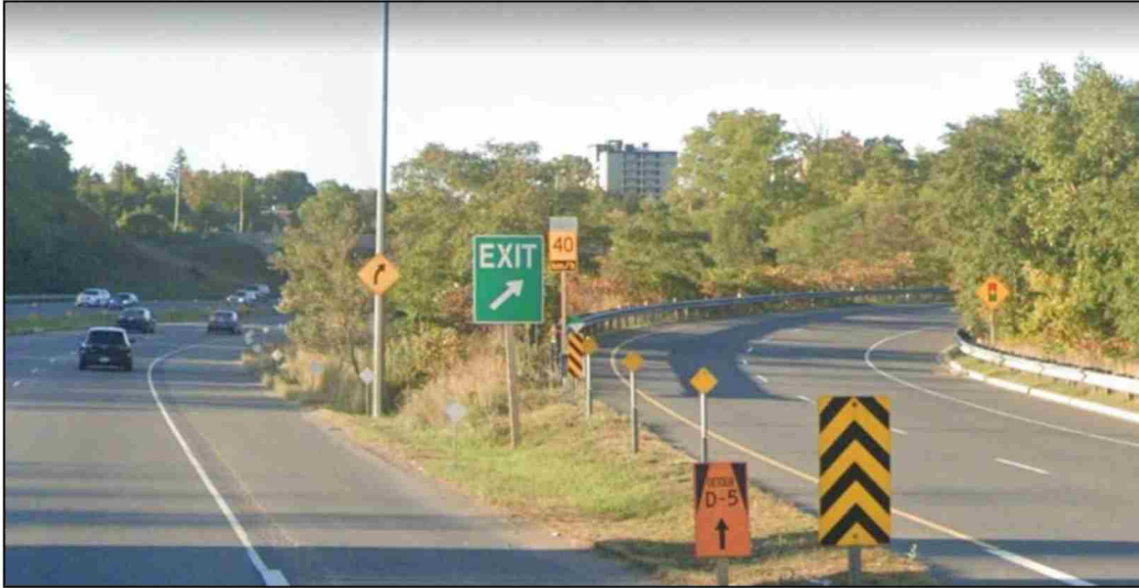
Figure 16: Southbound RHVP approaching the King Street (Google Maps, 2022).
