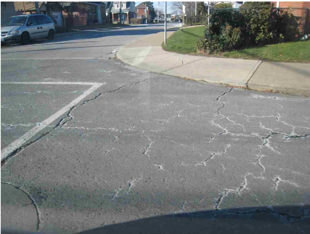
Typical Condition of Pavement Containing Steel Slag
