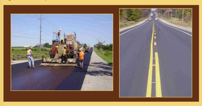
Micro Surfacing may be designed to correct rutting, improve inadequate pavement cross sections, seal minor cracking, and enhance frictional properties of structurally sound pavements.
