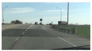
Figure 25 - Pole within Deflection Area of Approach Eccentric Loader End Treatment (View North from Beginning of Off-Ramp)
