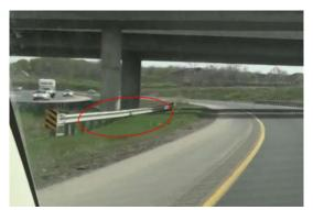
Figure 22 - Uneven Terrain Immediately In Front of the Steel Beam Guide Rail System (View North from the Mainline)
