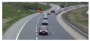
Figure 21 - Potentially Restricted Sightlines for Merging Traffic
