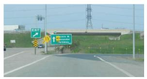
Figure 29 - Closely-Spaced and Eclipsing Signage (View West from Beginning of On-Ramp)
