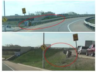
Figure 24 - Damaged and Poorly Designed Guide Rail End Treatment
