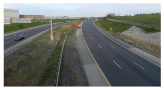
Figure 15 - View of Discontinuity in Horizontal Curve on the Mainline (View West from Pritchard Road Overpass)
