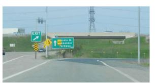
Figure 27, - Closely-Spaced and Eclipsing Signage (View West from Beginning of On-Ramp)
