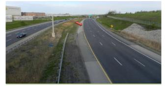
Figure 16,- View of Discontinuity in Horizontal Curve on the Mainline (View West from Pritchard Road
