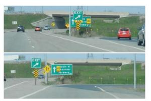
Figure <u>25</u>,- Closely-Spaced and Eclipsing Signage (View West from Beginning of On-Ramps)
