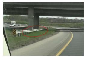
Figure 20,- Uneven Terrain Immediately In Front of the Steel Beam Guide Rail System (View North from the Mainline)
