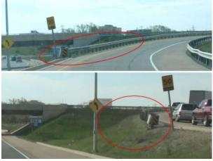
Figure 22 - Damaged and Poorly Designed Guide Rail End Treatment
