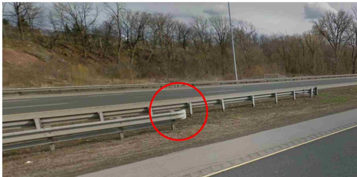
Figure 18: RHVP typical guide rail leaving end treatment
