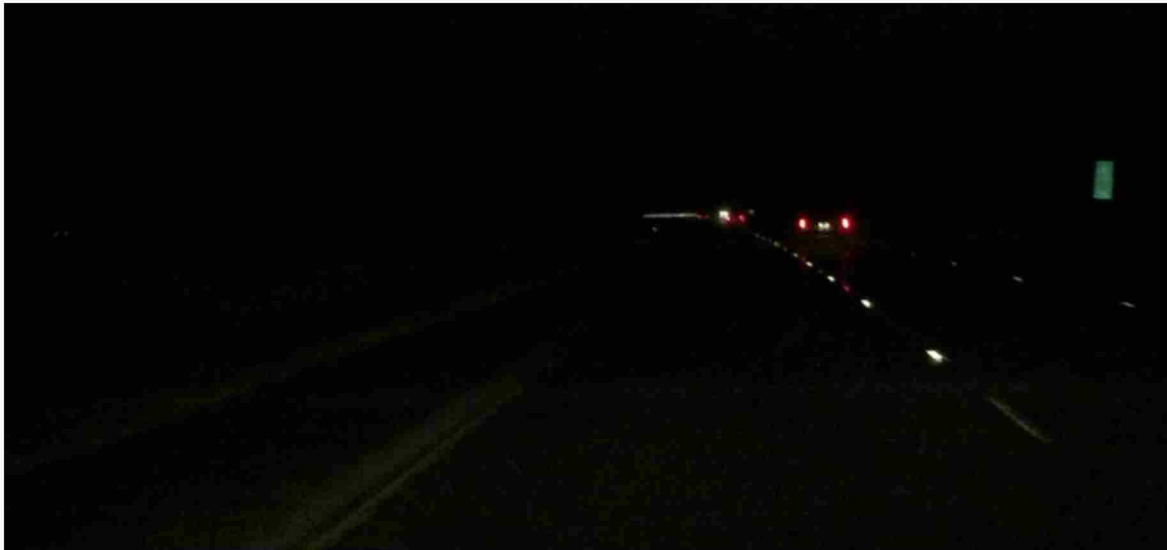
Figure 27: Pavement markings during nighttime condition (with PRPMs)
