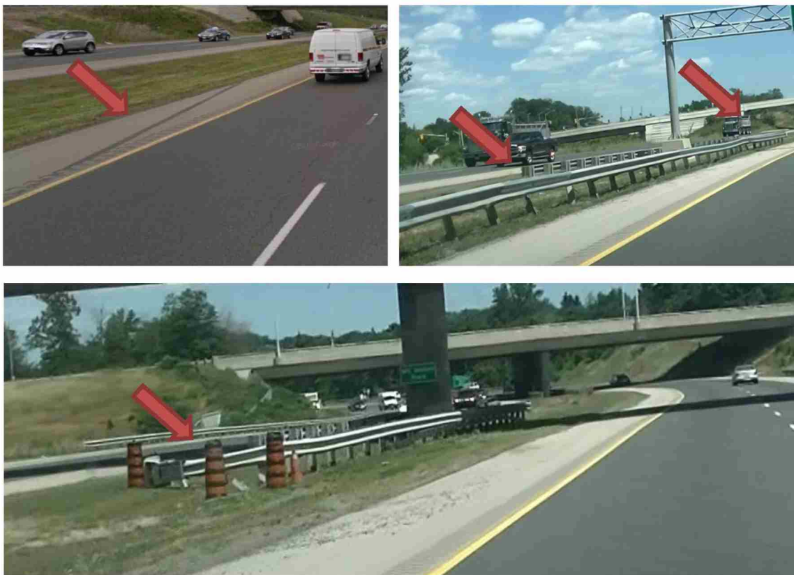
Figure 17: Evidence of loss of control towards the median / collisions with guide rails
