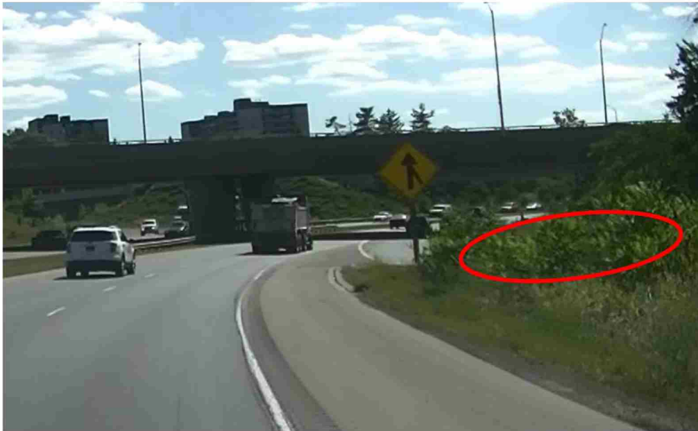
Figure 20: Vegetation obscuring view of vehicles approaching from on-ramp
