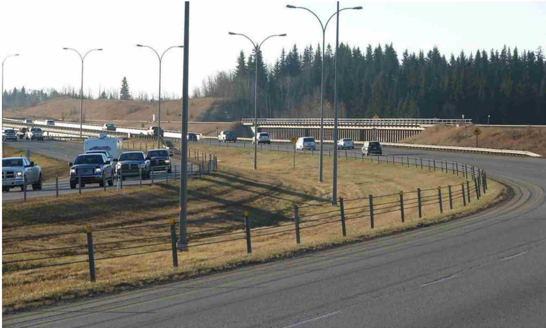
Figure 31: Example of high tension cable barrier
