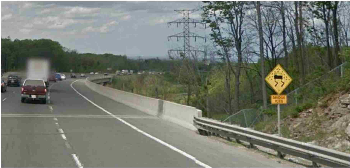
Figure 22: SLIPPERY WHEN WET sign + BRIDGE ICES tab sign
