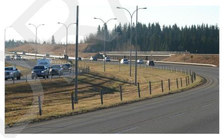
Figure 2: An Example High Tension Cable Barrier
