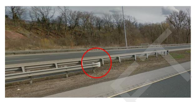
Figure 18: RHVP typical guide rail leaving end treatment
