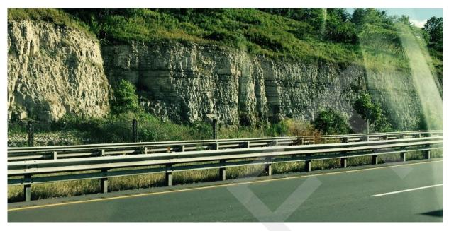
Figure 30: Example of standard steel beam guide rail with channel
