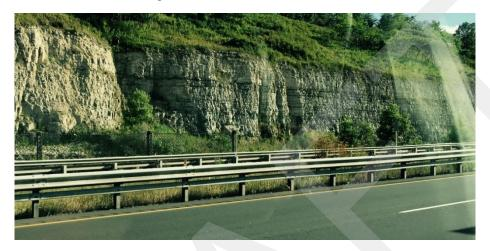
Figure 1: An Example Standard Steel Beam Guide Rail with Channel System
